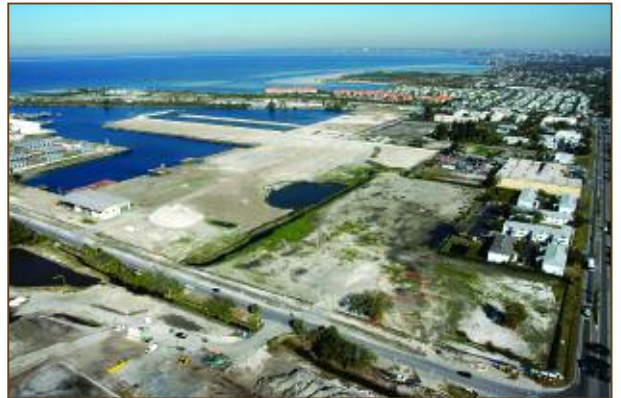
'After' aerial photo of dismantled area
