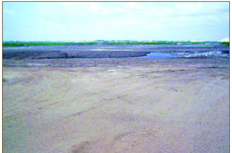
Cleared site ready for mining
